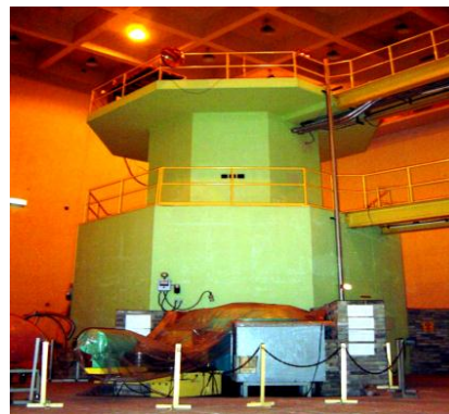
Fig. 1. The TRIGA reactor shield structure [26].
